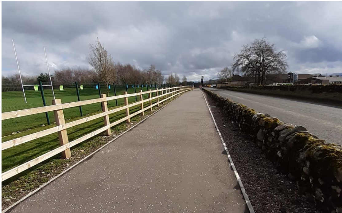
Figure 12: The new footpath involved purchasing land behind the wall to build a new footway and make the connection from the Crieff Primary and High Schools, Community Centre and Library, skatepark, and sports fields past the new shopping superstore development and back towards town (Image © Perth & Kinross Council)
