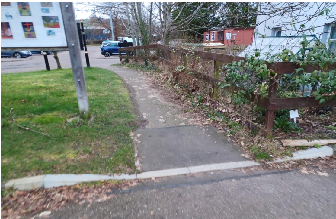
Figure 9: A new drop kerb at a well-used cut through to the shops and schools in Dingwall (Image © Highland Council)
