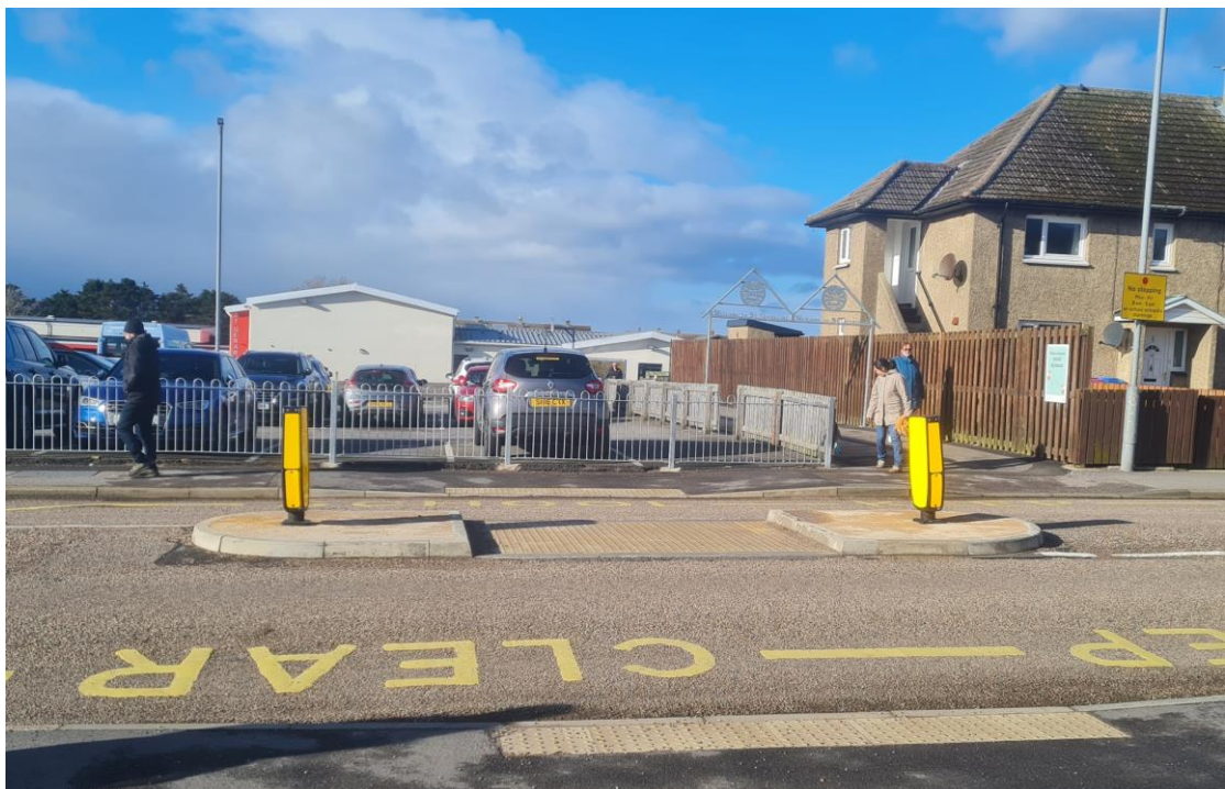
Figure 15: The new crossing island in front of the main entrance of St Geraldines Primary School was identified in the School Route Audit in Lossiemouth (Image © Moray Council)
