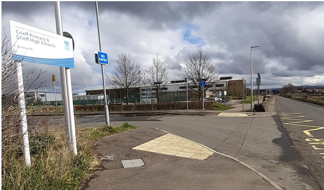
Figure 2: Drop kerb and tactiles were the second most frequently identified community recommendation, but only two local authorities delivered on these (Image © Perth & Kinross Council)
