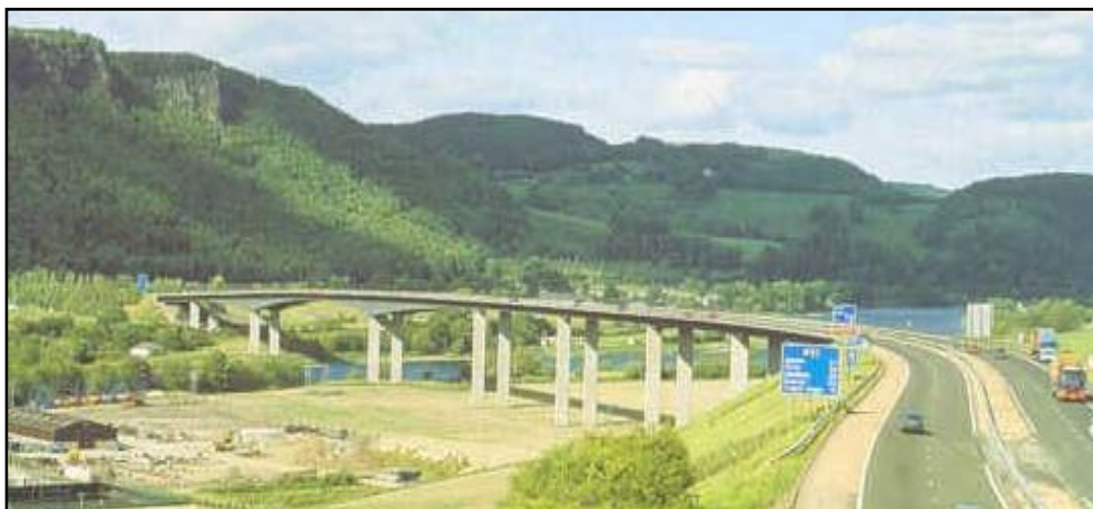
Figure 4.15.2.A – M90 10-11 55 Friarton Bridge
