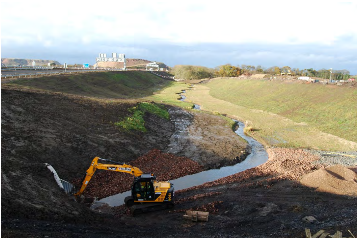
Realignment of previously canalised Swine Burn to return it to a more naturalistic and ecologically healthy state at Junction 1A on the M9 as part of the Queensferry Crossing Project.
