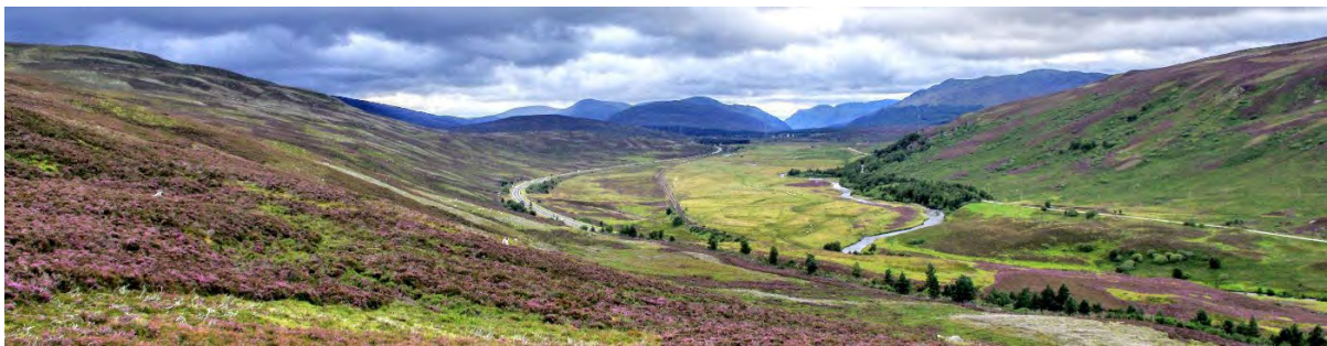
The A9 and Highland Mainline Railway, passing through ecologically sensitive upland landscape Photo: Jacobs/Gareth Talbot
