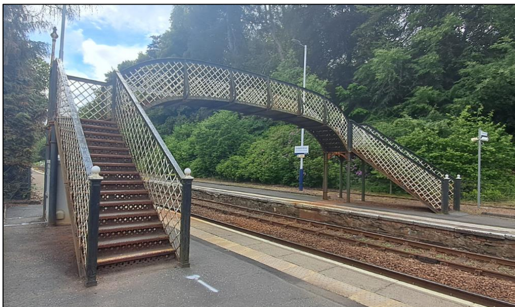
Photograph 9.4: View of the cast-iron footbridge located to the south-east of the station and forming part of Asset 26, facing south-east. Jacobs, 2024.
