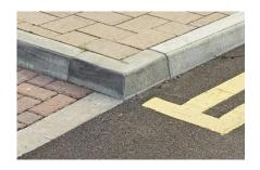
A **kerb** separates areas that are used for by different things, like separating walking and cycling, or walking and cars.
